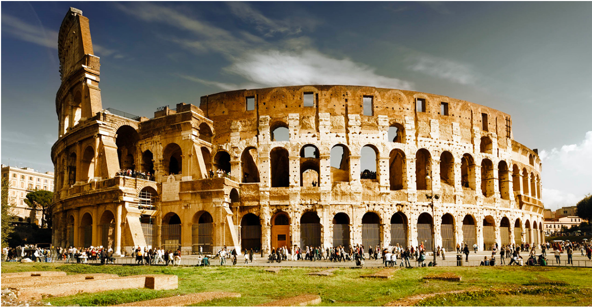
Coliseum. Rome, Italy. Built of travertine limestone, tuff (volcanic rock), and brick-faced concrete. https://gharpedia.com/blog/mysterious-roman-concrete-standing-for-2000-years/
