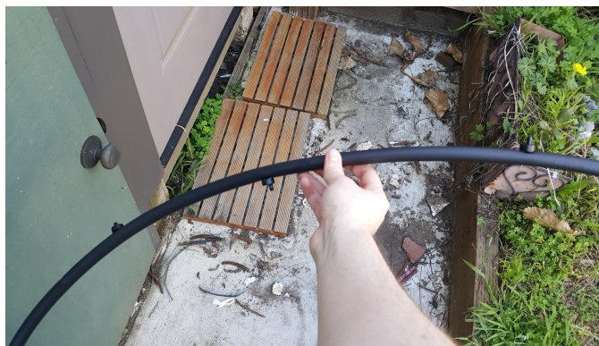
Fig. 9: Branch tube with drip valves
