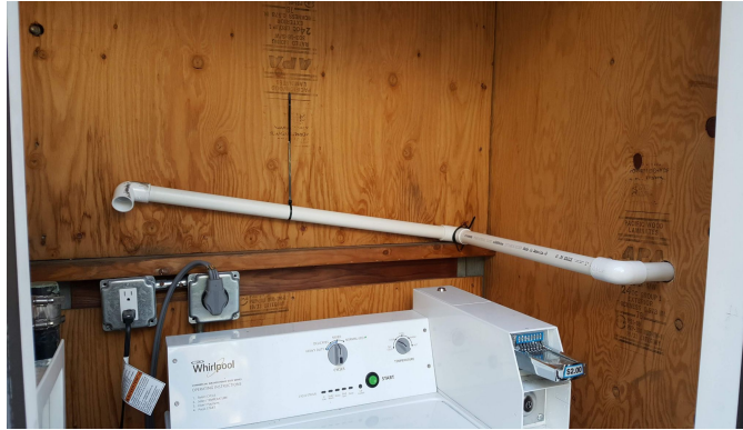
Fig. 5: Sealed and installed piping. Notice downslope for water movement
