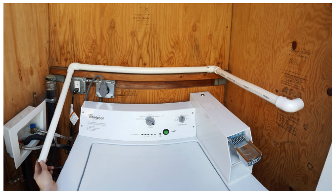
Fig. 4: Dry fit inside the washing machine closet
