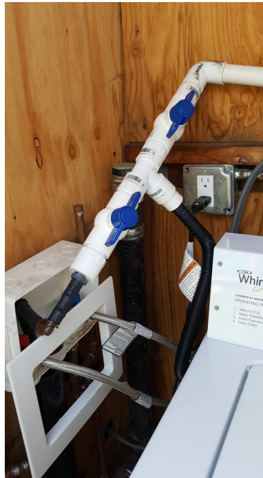
Fig. 15: Completed T-valve system
