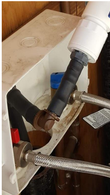
Fig. 14: Irrigation tubing with L-joints to maneuver into the sewer pipe
