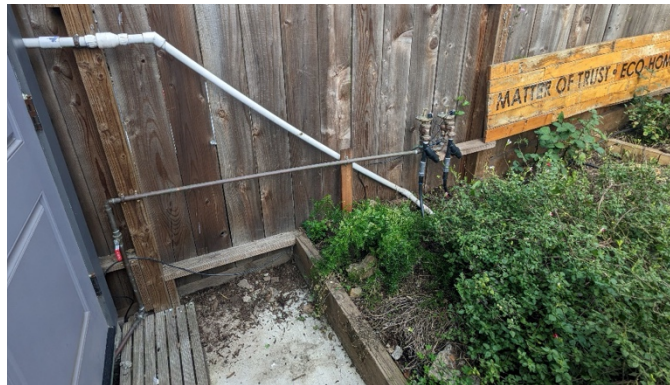
Fig. 20: Laundry to Landscape tubing (white), along with the new irrigation system (copper pipes)
