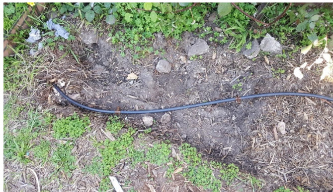
Fig. 8: Main "trunk" tube with T-joints
