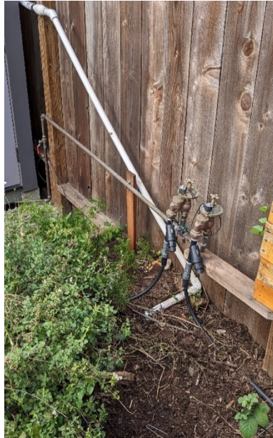
Fig. 17: New graywater outflow into garden
