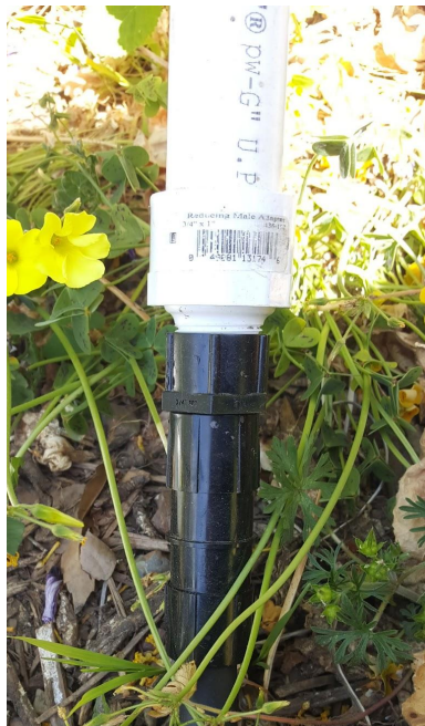
Fig. 11: PVC to irrigation connection
