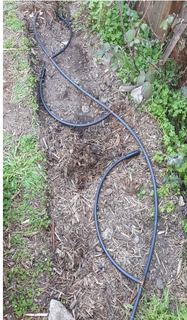
Fig. 10: Branch tubes attached and capped
