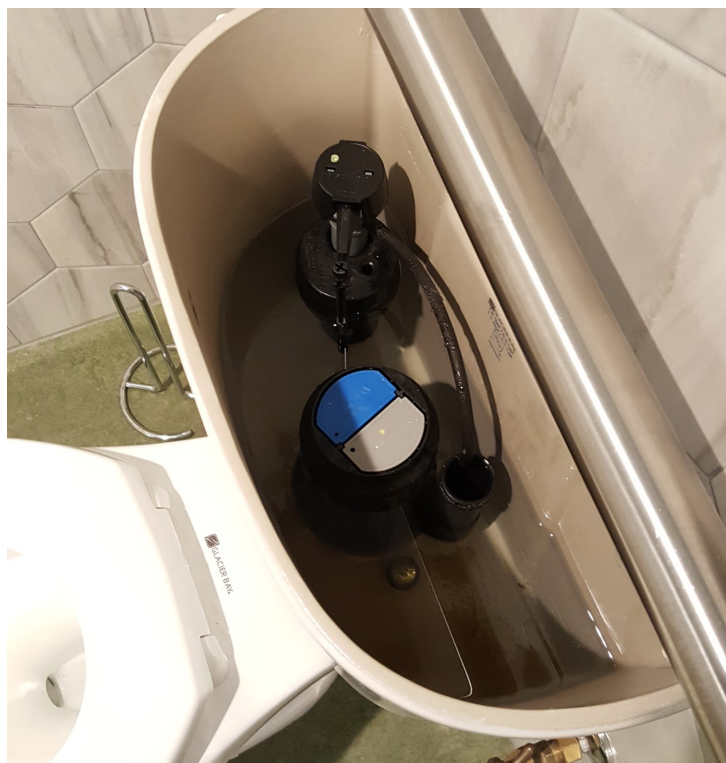
Fig. 2: Centered flushing mechanism (blue and gray cylinder)
