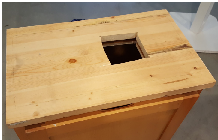
Fig. 5: Wood panel installed and holes cut for sink drain
