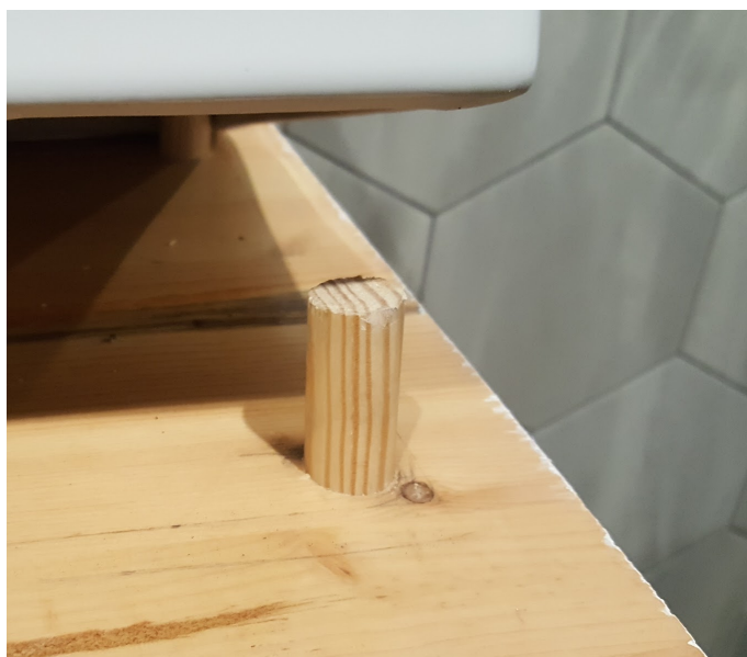
Fig. 6: Dowel rods used to keep the sink in place
