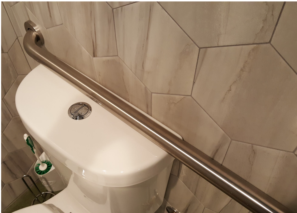
Fig. 1: Centered flushing mechanism & ADA bar
