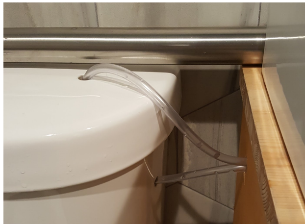
Fig. 13: Sink tubing threaded into the tank
