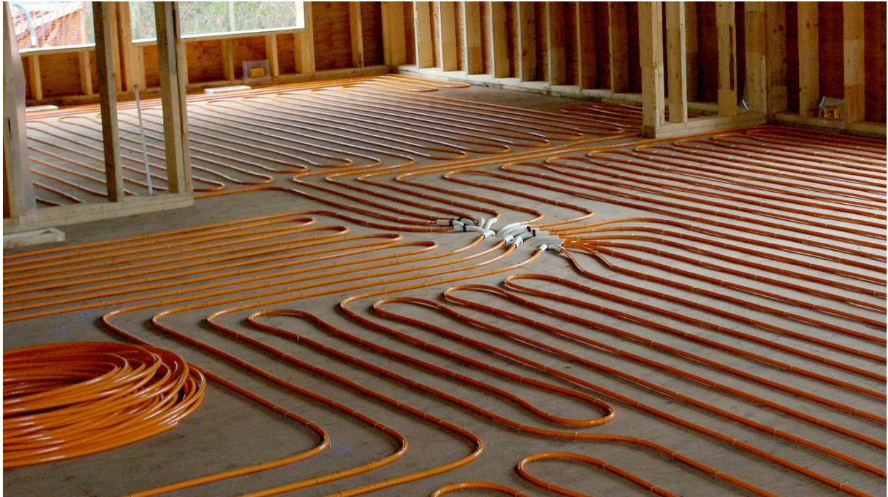
An example of hydronic radiant heating - image via tingeypumbing.com
