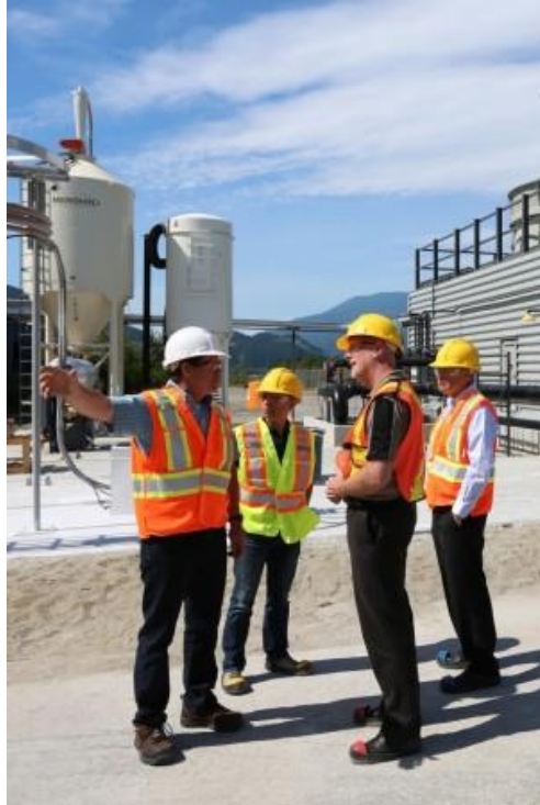
Carbon Engineering's demonstration project in Squamish, B.C. will be capable of scrubbing 2 tons of CO2 from the air daily. PHOTO: Carbon Engineering
