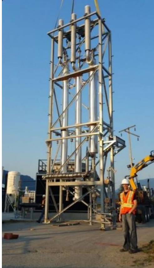
Construction underway at the Squamish facility. PHOTO: Carbon Engineering
