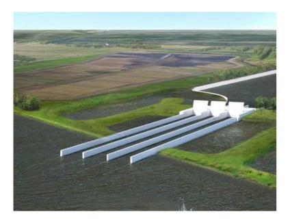
Sediment diversions mimic nature's historic land-building processes by using the power of the river to move sediment and fresh water into nearby basins. This project type can build new land and is critical for helping sustain new and existing wetlands. Sediment diversions provide a sustainable source of sand and mud over time to sustain nearby marsh creation, barrier island and ridge restoration projects.
