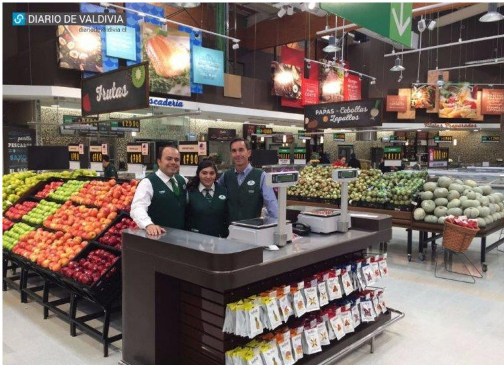
Staff at the Jumbo supermarket in Valdivia, Chile. The new supermarket is using transcritical CO2 for its refrigeration
