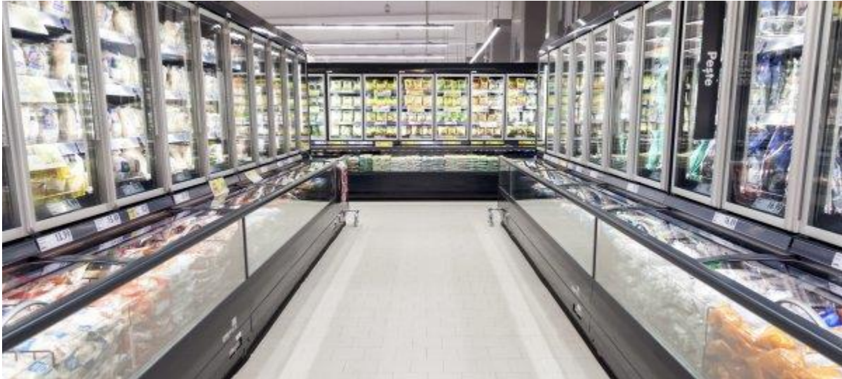
Jumbo supermarket in Valdivia, Chile installs transcritical carbon dioxide refrigeration
