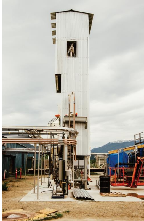
Dried pellets are fed into the calciner, in which a 900 °C inferno of natural gas burning in pure oxygen roasts a rolling mass of calcium oxide. The calcium carbonate pellets spontaneously break down, producing more calcium oxide and releasing carbon dioxide gas.
