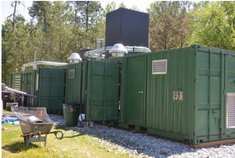
The Battalion-scale Waste to Energy Conversion Green Energy Machine converts 3 tons of trash into 100 gross kilowatts of energy. (Photo Credit: Danielle Davis)
