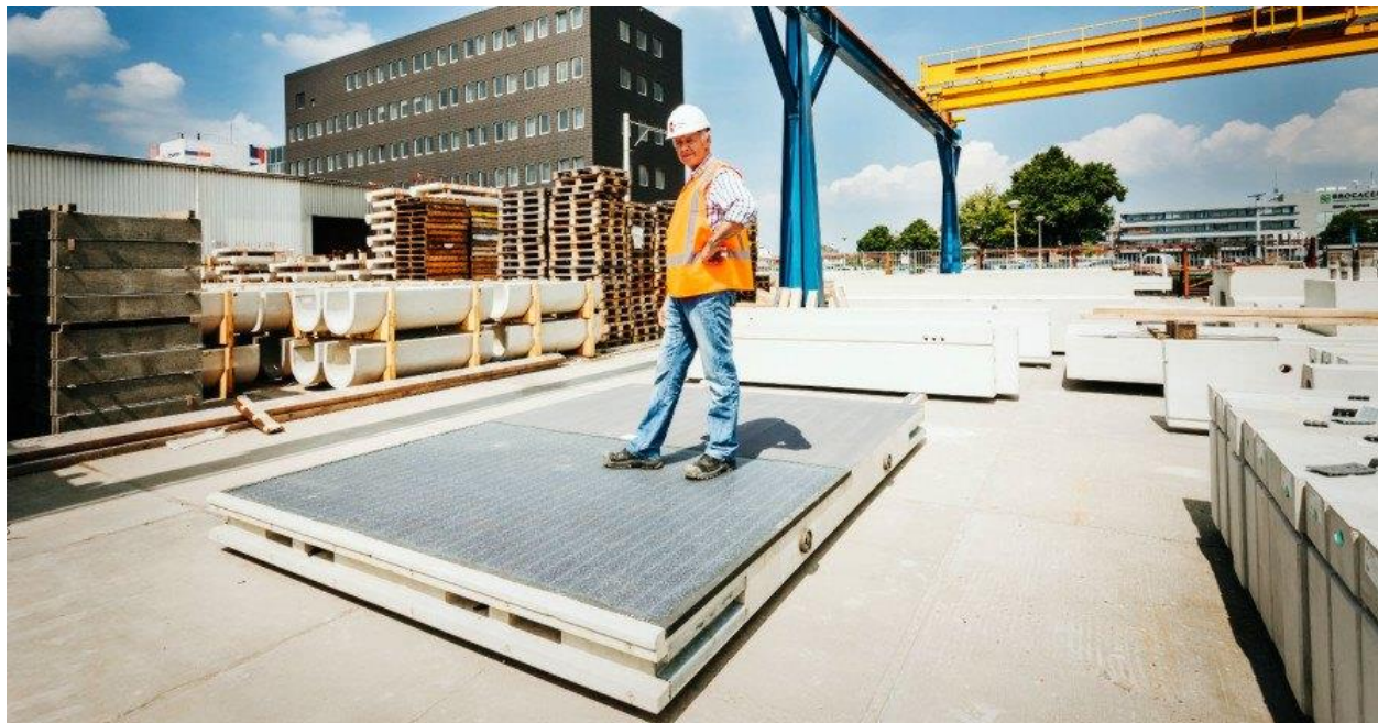
SolaRoad Netherlands Solar Sidewalk Construction
