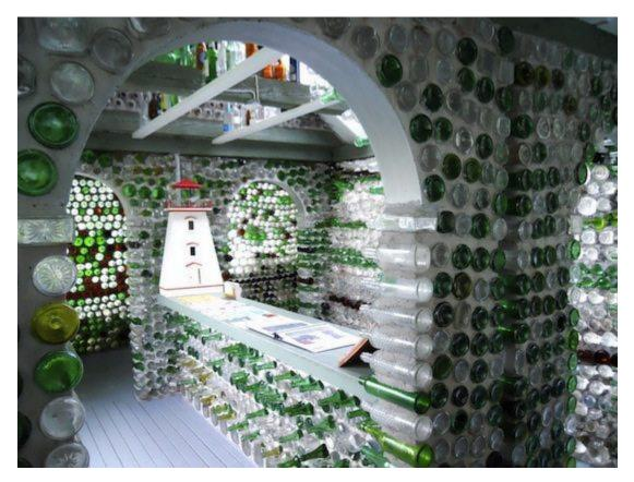
The first glass house that Édouard built was a six gabled house. This house has three main sections and measures 20 ft x 14 ft. This house has incredible patterns resulting from the careful selection of bottle colours and sizes. To create the look, Mr. Arsenault cemented between 300-400 bottles per row. This glass bottle house was built over a six month period. Approximately 12,000 bottles and 85 bags of cement were used.
