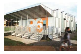
The structure is topped with a distinctive sawtooth roof that uses north-facing windows to optimize ventilation and natural daylight to the interior.
