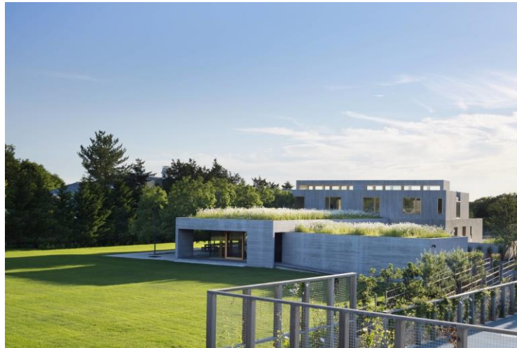
Photo: Michael Moran/OTTO for Andrew Berman Architect
