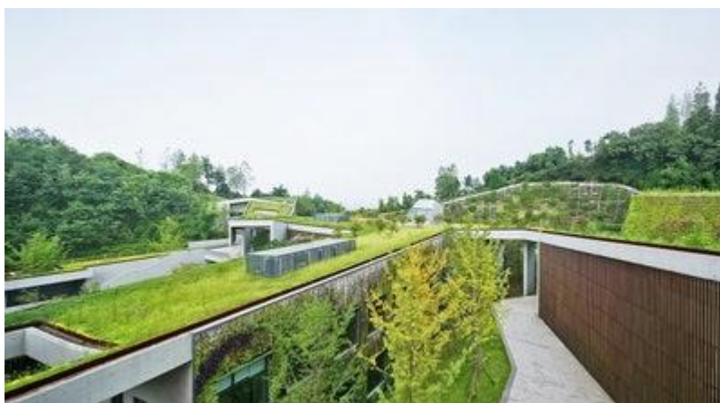
Photo: Courtesy of Vector Architects 5/16
