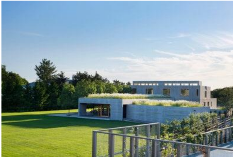
Photo: Michael Moran/OTTO for Andrew Berman Architect 1/16
