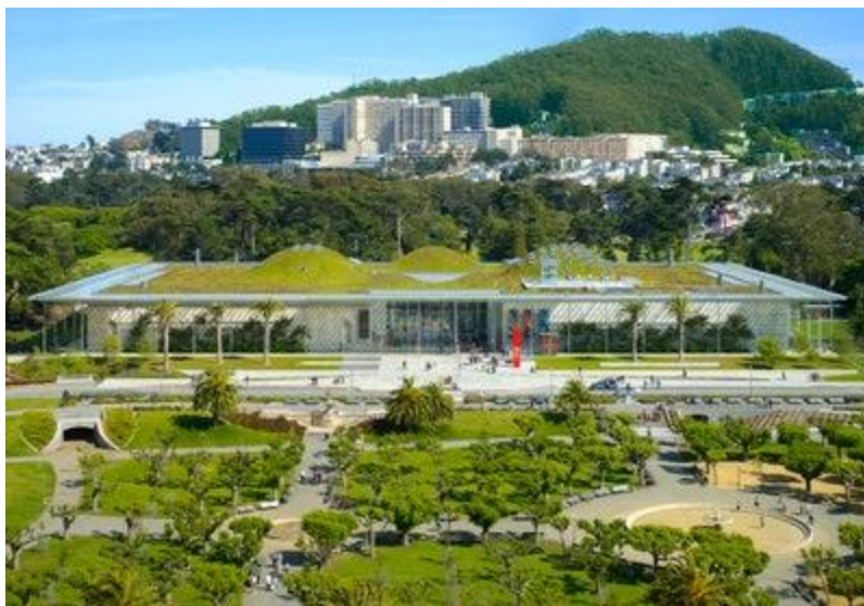
Photo: Tim Griffith 12/16
