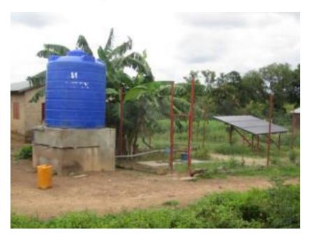
Solar panels also power the water pump to supply water for domestic use. This reservoir is connected to six water taps. (image via Chad Lipton/National Geographic Society)
