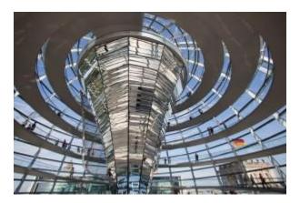
The Reichstag, Germany's parliament building, was retrofitted in 1999 with a new dome that uses glass and mirrors to reflect daylight deep into the main chamber, reducing dependence on artificial lighting. It also employs a funnel to divert and collect rainwater.
